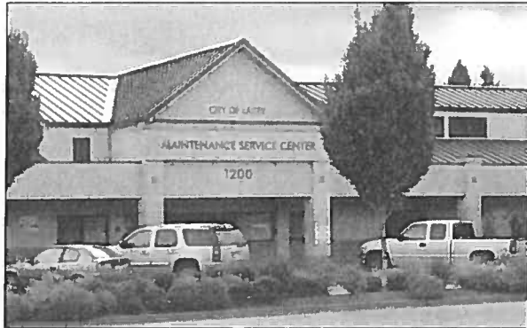
The City of Lacey, Washington, owns and operates three different types of wastewater collection systems: gravity, STEP, and grinder.
